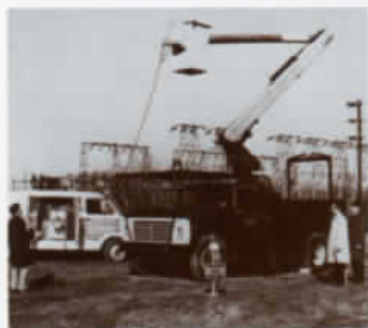
Mobile High-Voltage Testing
