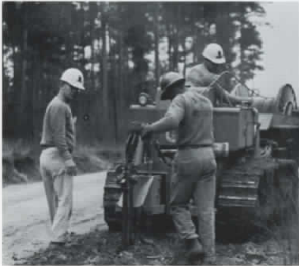
Asplundh Service Company crew, trenching and cable-laying
