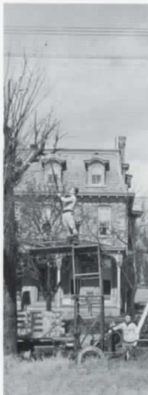
Asplundh platform lift was elevated by a hand-cranked system. This was the company's first attempt at mechanizing its operations.
