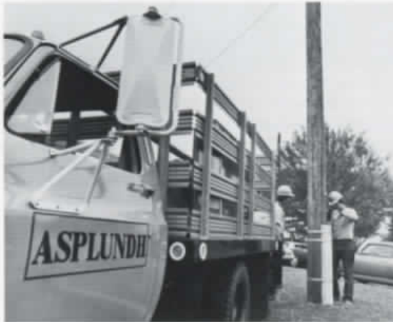
Reinforced distribution pole after installation of steel-beam support.
