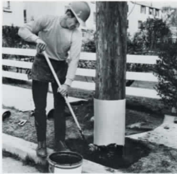
Application of the "Pole-Tox" pole preservative
