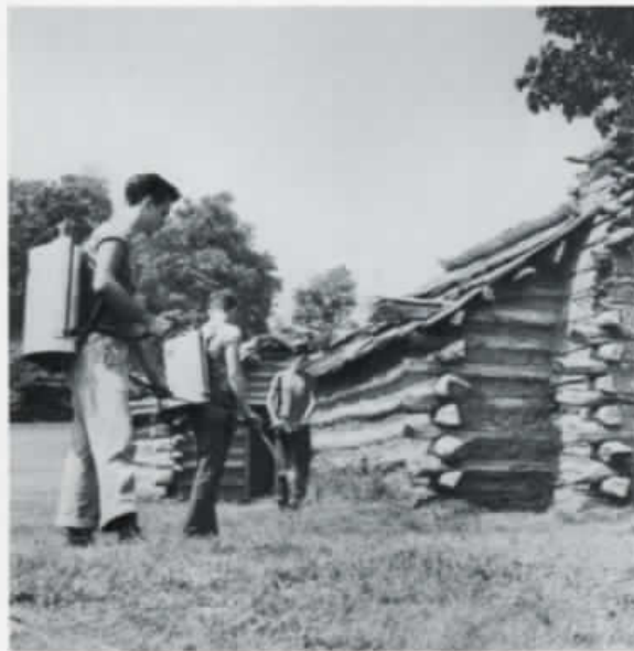
Chemical spray operations at Valley Forge Park
