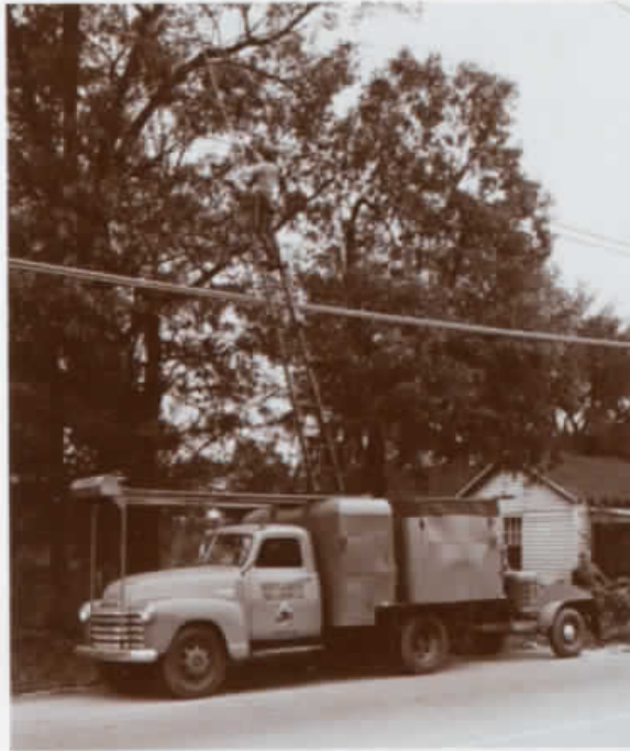
Wooden ladders were mounted on revolving turrets to allow the trimmers better access to the trees.
