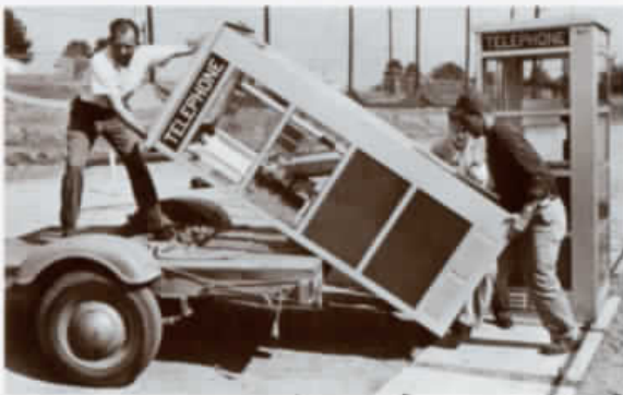
Phone booth installation and maintenance were the first operations of the Asplundh Service Company
