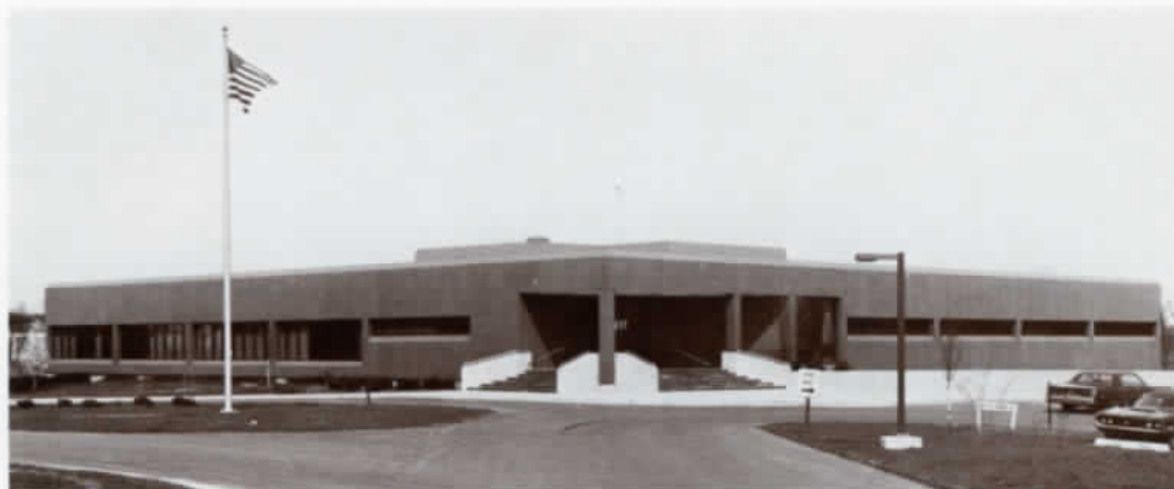
Asplundh's new headquarters at Blair Mill Road, Willow Grove, Pennsylvania.
