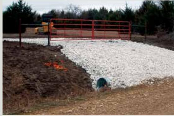
ABC is well-equipped to install gates and fencing for utility access and protection of livestock. ABC also builds rock road entrances to rights-of-way to keep public roads clean and prevent damage from heavy equipment use.
