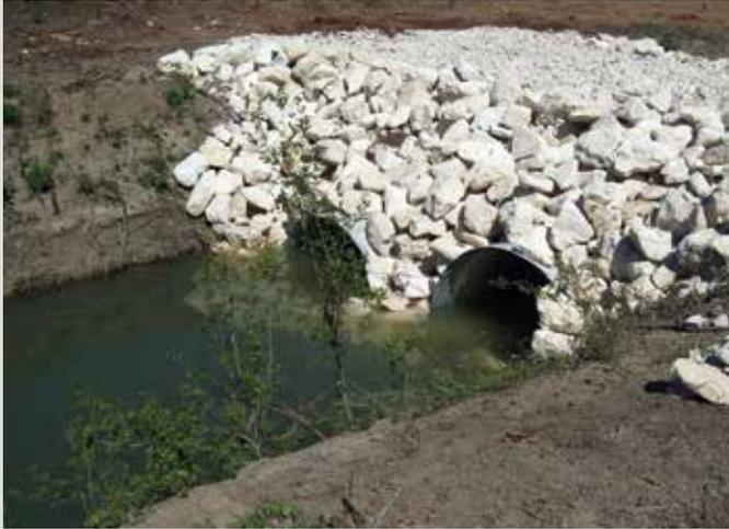
Access road and work site construction often requires installation of culverts, as well as moving large volumes of material to protect streams and wetlands.
